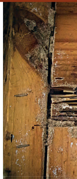
This garage header beam has such an active termite infestation that a pen easily slips through.
